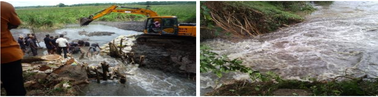
Eppawala tank damage
