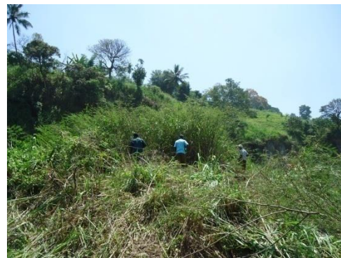
figure 1.1.9 – Clearing of excessive growth (Sangilipalama- Kothmale)
