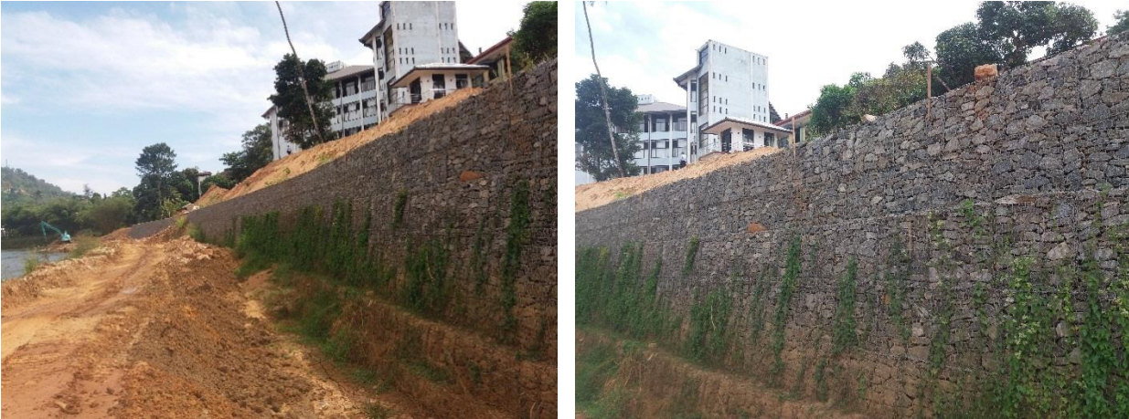
Construction of gabion wall at river bank of Mahaweli - Gatambe
