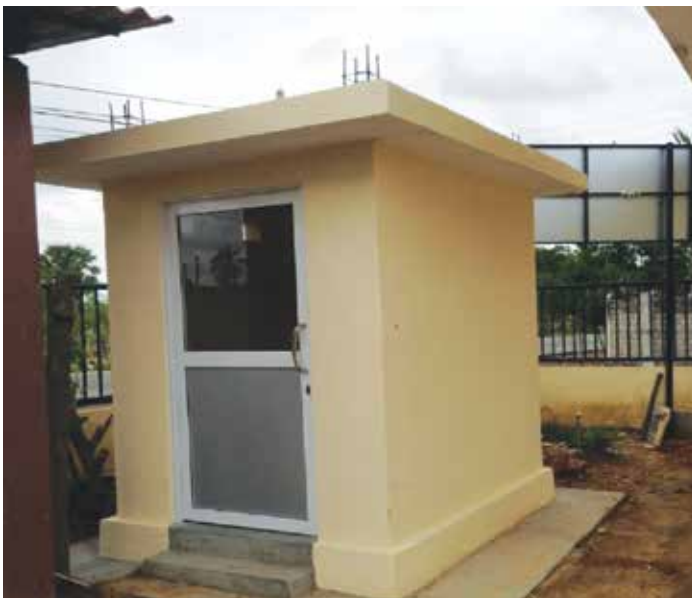
Renovation of Computer Room at ATI Kandy
