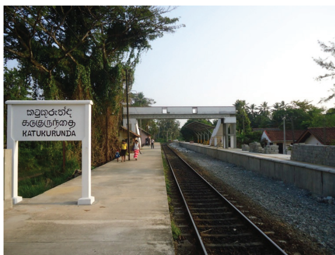
Construction of double line from Kaluthara South to Payagala South overhead bridges, platform and railway station
