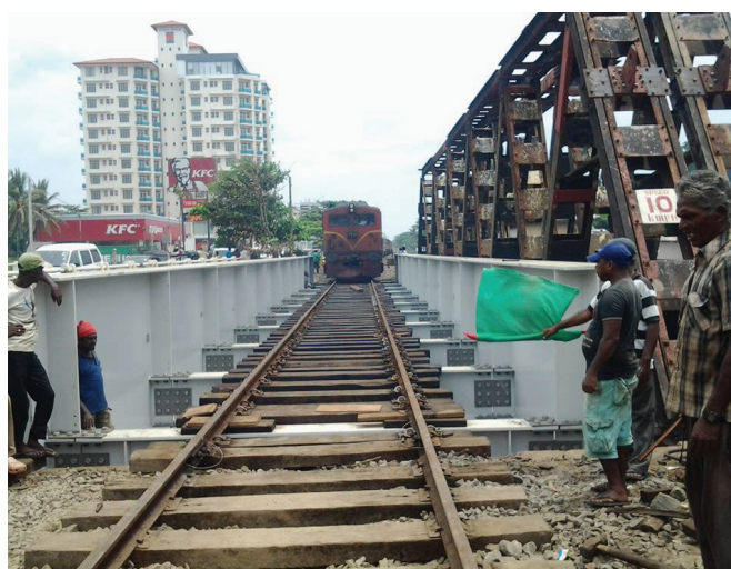
Replaced bridges at Wellawatta under the Belgium line of credit
