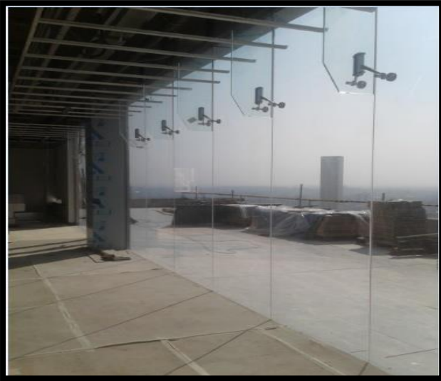
Roof Terrace Kitchen fixing Glass windows
