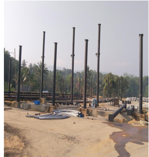
Construction of weekly faire Nivithigala
