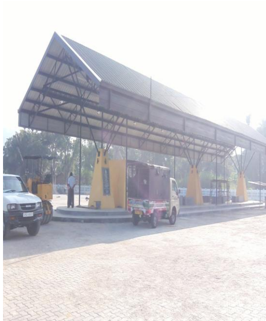
Construction of bus-stop Nivithigala
