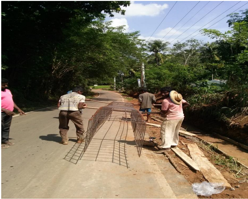
Carpetting Udawalawa South bank road
