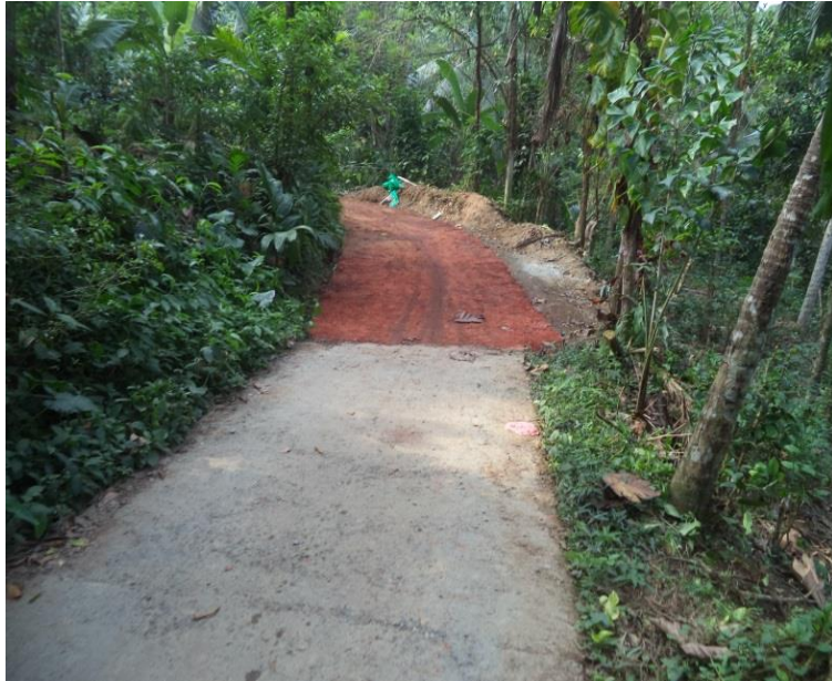
Post 40, Wellambura road
