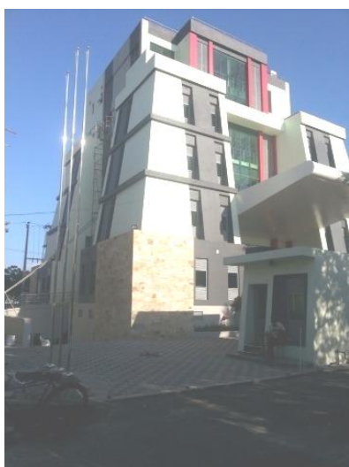
AGM Building at Pannai
