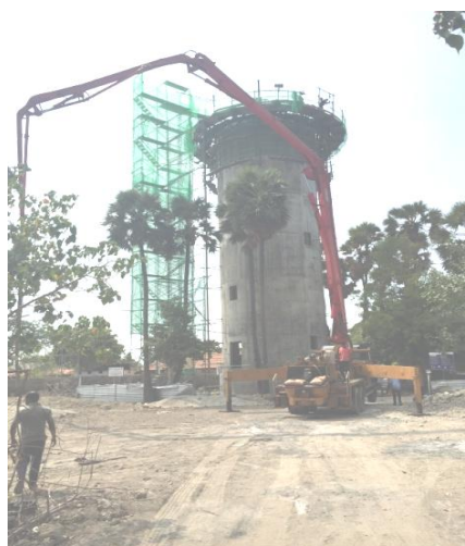
Water Tower at Punguduthivu
