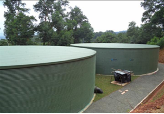
Ground Reservoir at New Town
