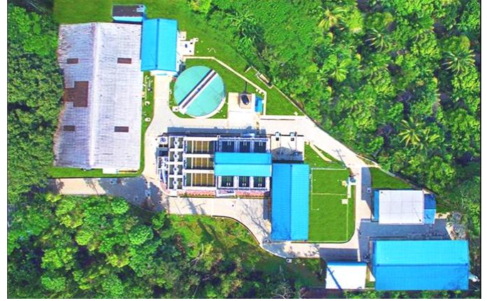
Water Treatment Plant & Pumping Station at Pompakele
