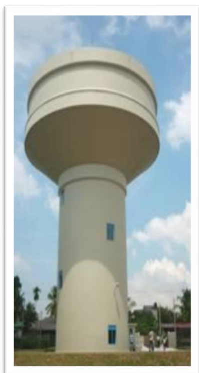
Water Tank at Kesbewa
