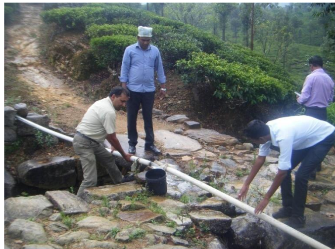
Repair of water sources in the Estate Sector
