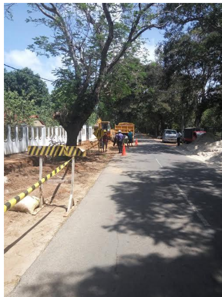
Pump laying for sewerage –02 Zone Sella Road
