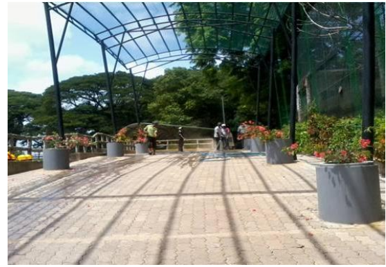
Construction of internal roads -Dehiwala
