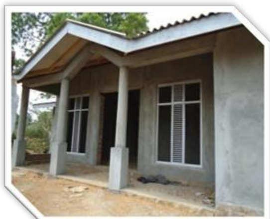
Expansion of laboratory building of Arthur C. Clarke Institute, Katubedda
