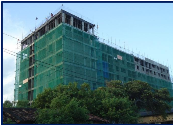
Angulana Housing Project in Progress
