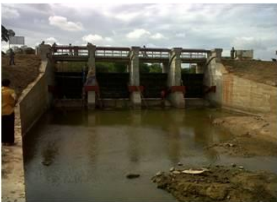
Fabrication and installation of 4 sluice gates- Ellapathana project
