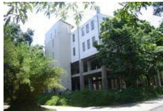
Department of Textiles -Moratuwa University building
