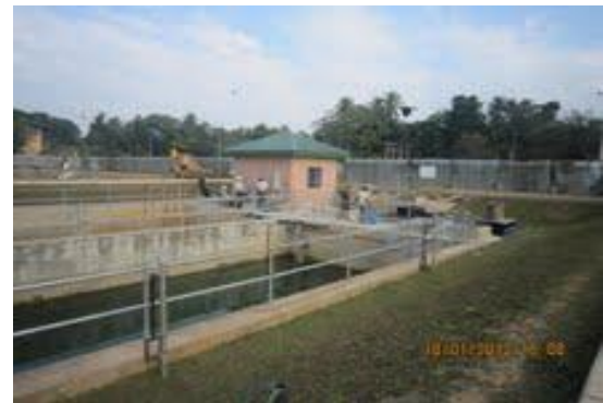
Water treatment plant- Katugastota
