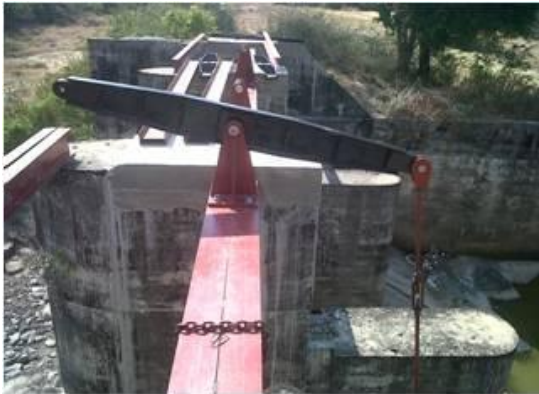
Fabrication and installation of 3 flap gates for Nelu Oya anicut
