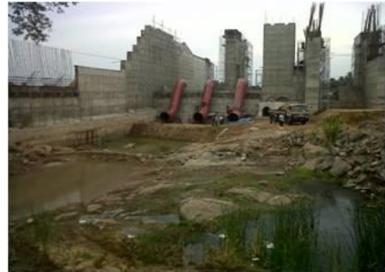
Fabrication and installation of 3 penstock pipes for small power plant being constructed at Deduru Oya reservoir
