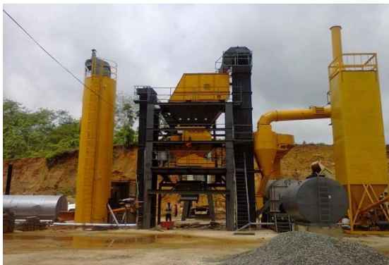
Plant manufacturing asphalt mixture for road carpeting
