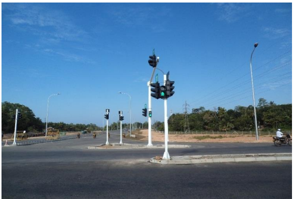
Installing traffic light systems Godagama, Matara
