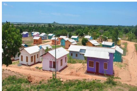
Periyakulama housing project
