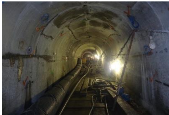
Tunnel at the New Laxapana power station
