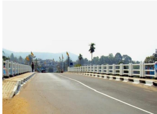
Ruwanwella bridge project
