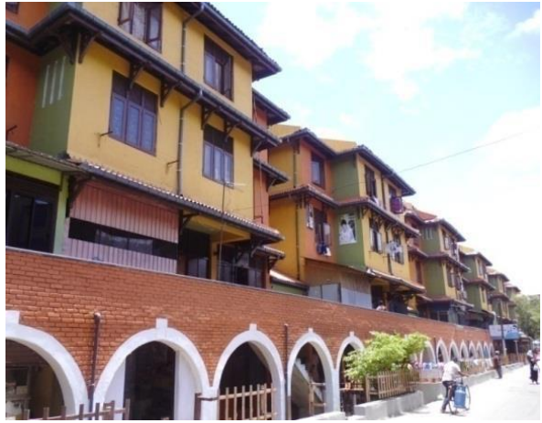
Gunasinhapura housing project
