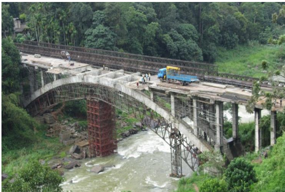
Construction of Ulapane bridge
