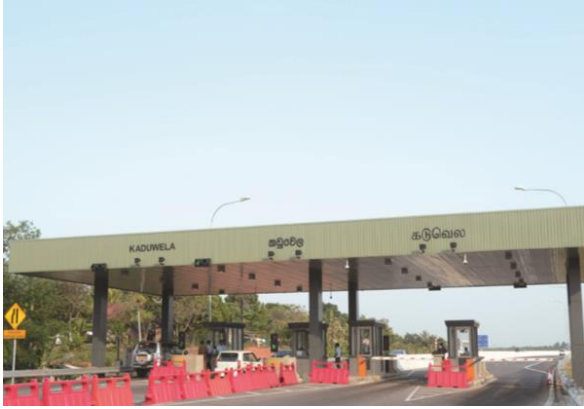
Kaduwela expressway entry point building
