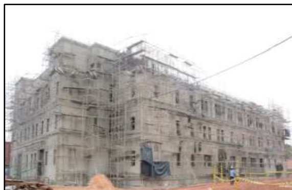
Communication Building and Signal Tower
