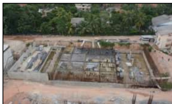
Water Sump and Pump House
