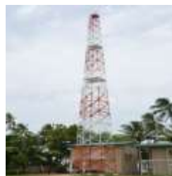
40 m Communication mast at SLCG Rohana Life Saving points in Morogolla and Unawatuna
