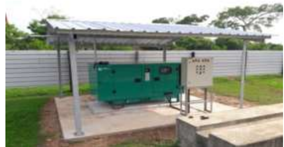
Generator installation at Kokavil
