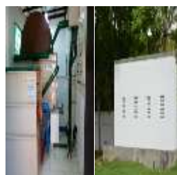
Sewage Treatment plant at SLCG Rohana
