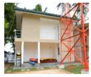
Coast Guard Operations Room, PABX and utility complex
