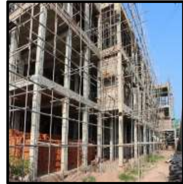
Progress up to 31 st December 2016.
