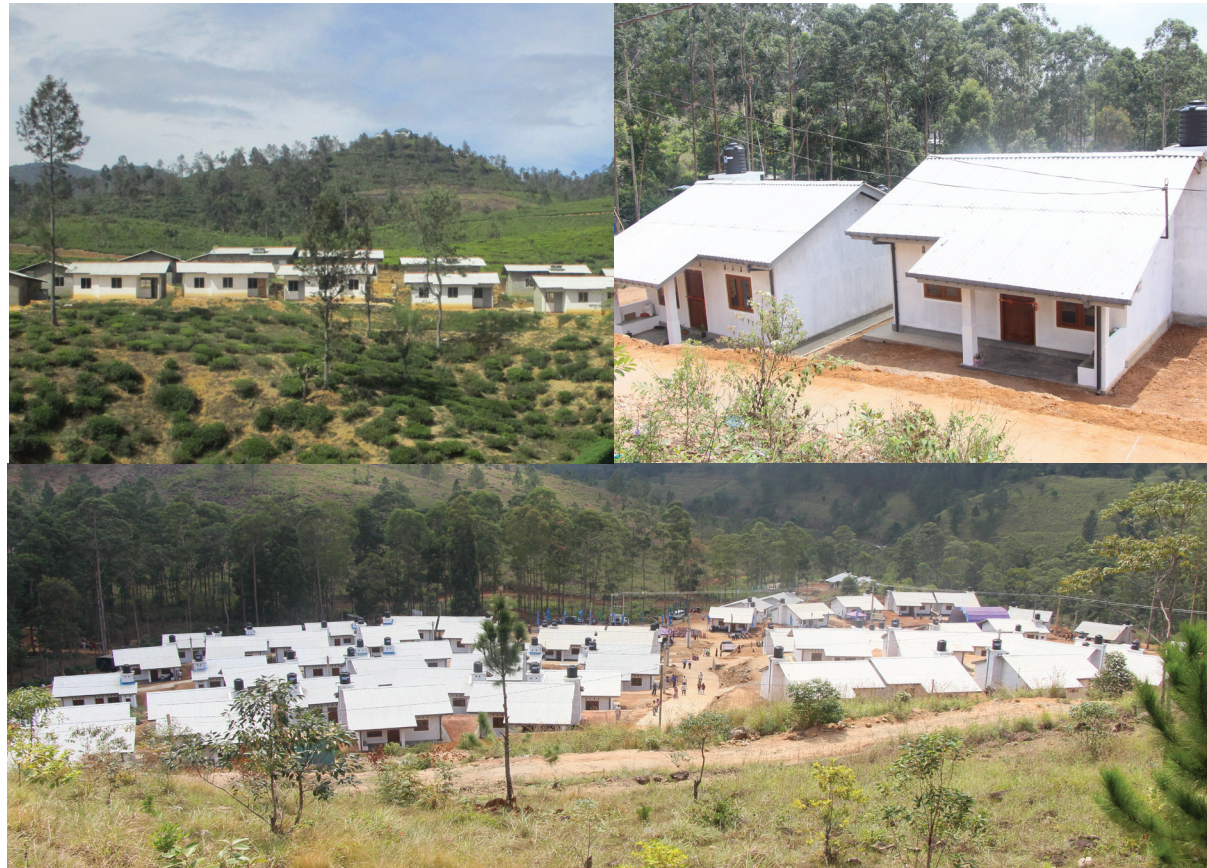
Housing Project implemented by Rathnapura Regional office, at Doloswala Estate, Kolombagama Division in Agalawatta Plantation Company Beneficiaries - 30 Families, Estimated Cost - Rs. 36 Mn
