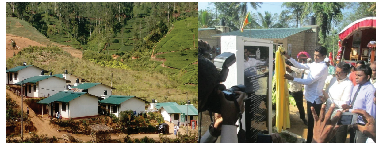
Housing Project implemented by NuwaraEliya Regional office, at Albian Estate, Aldlaw Wedamulla Division in Agarapatana Plantation Company Beneficiaries - 10 Families, Estimated Cost - Rs. 6.5 Mn
