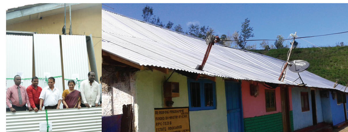
Re - Roofing Project Implemented by Kandy Regional Office at Rockwood Estate, Line Room No. 04 in JEDB Plantation Company
