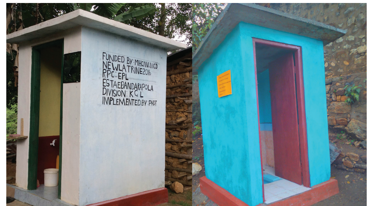
Latrine project implemented by Kegalle Regional office, at Adurapola Estate, Adurapola Division in Alptiya Plantation Company No of Units -10, Project Cost - Rs. 0.5 Mn
